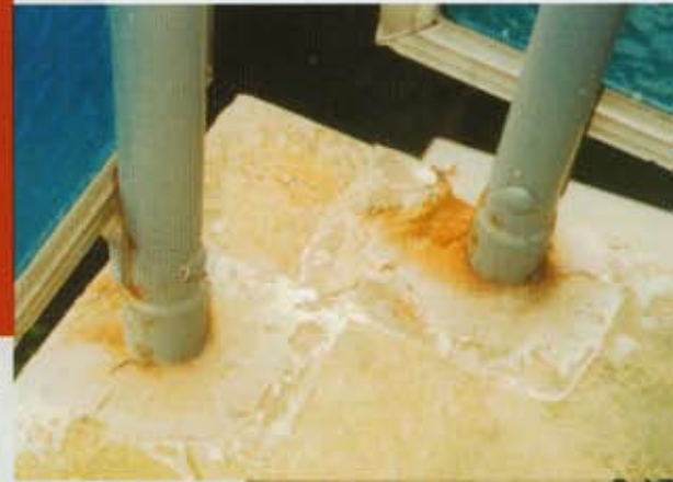
Handrail anchor repairs ▼
